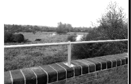
A beautiful view from part of the new Hockley Viaduct.
