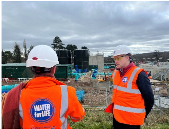
Steve at Southern Water’s water supply works at Otterbourne
